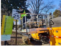
Image: Installation of new 25 mph signage Credit: ATLDOT
